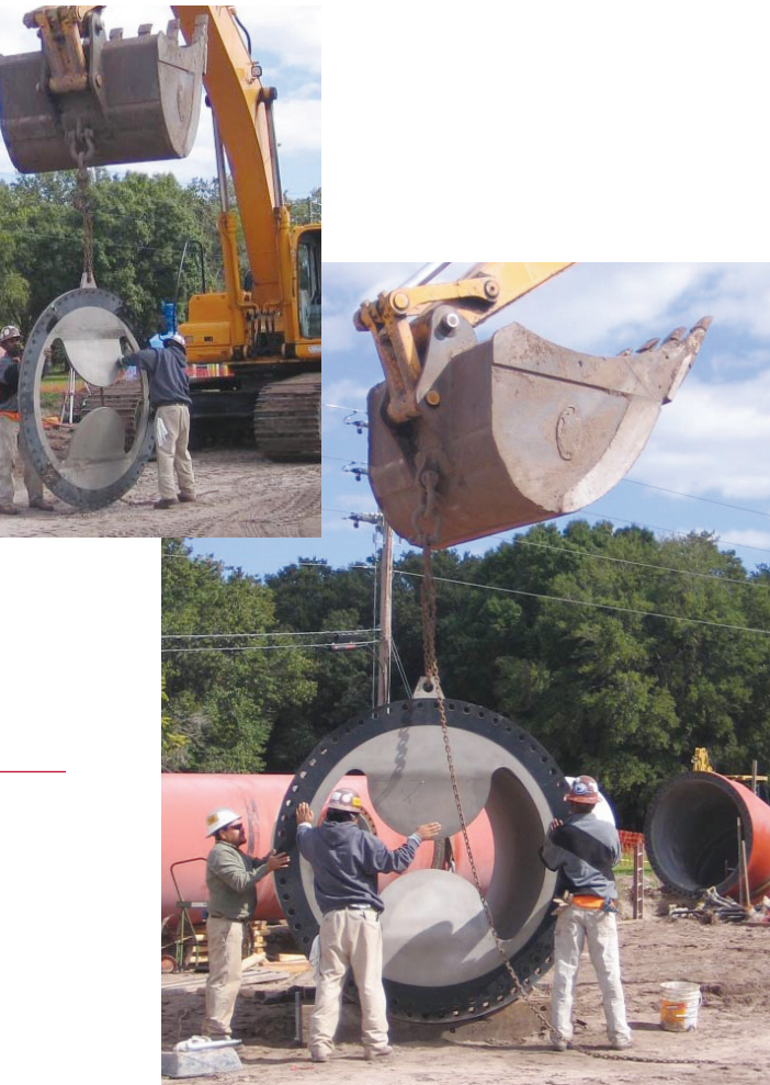
The mixer arrived with pre-applied gasket and pre-drilled flange for easy installation.
